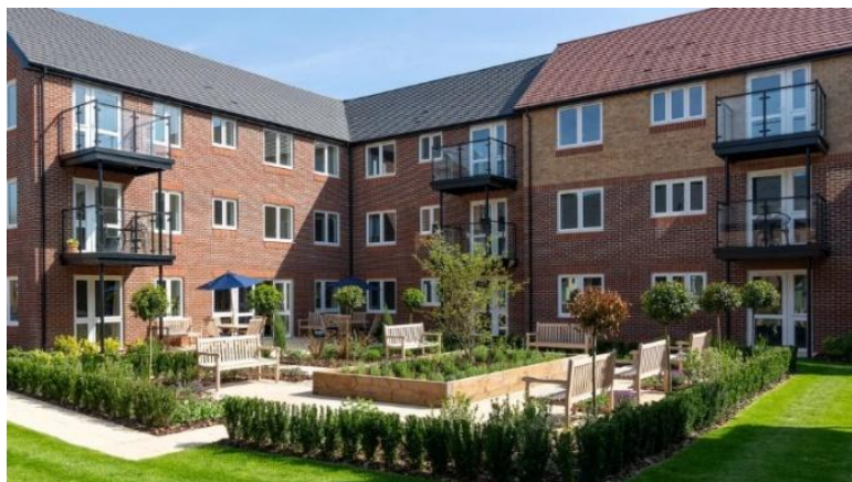
Figure 9.3 – Charles Lodge, Evesham
